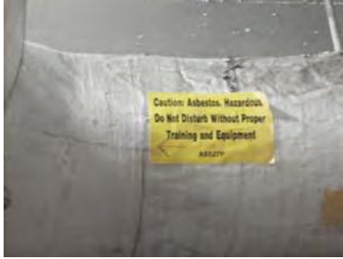
Asbestos insulation
