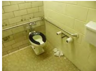
Plumbing fixtures to be replaced
